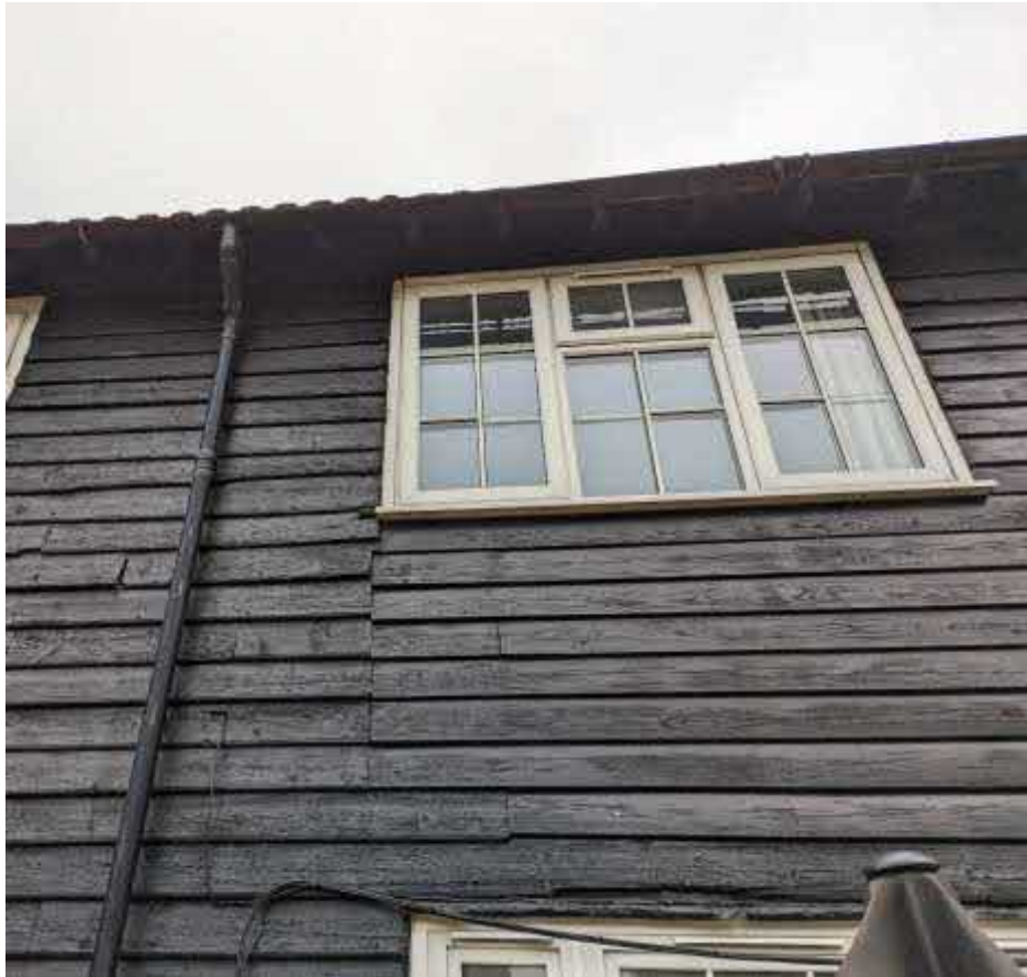
Fig.11: Prominent woodgrain of existing timber weatherboard cladding
