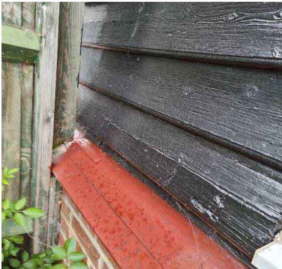
Fig.10: Prominent woodgrain of existing timber weatherboarded cladding
