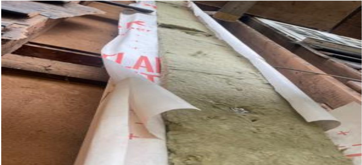
Fire stopping material installed between the properties prior to cladding replacement
