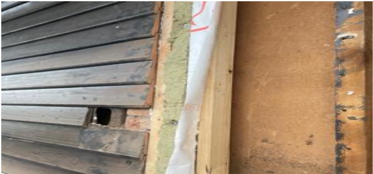
Cut back detail of the brickwork party wall line, this image shows the masonry, spanning the two properties. Board removed from freeholder side for illustration.
